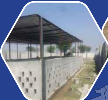
IRRC FECHS Under construction
